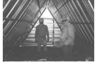
Each panel is braced with three 1-in. sq. tubing cross members.
