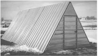
Shelter is constructed of 8 by 10-ft. panels that pin together, allowing two men to set up or take down an 11 by 24-ft. structure in only 30 minutes.
